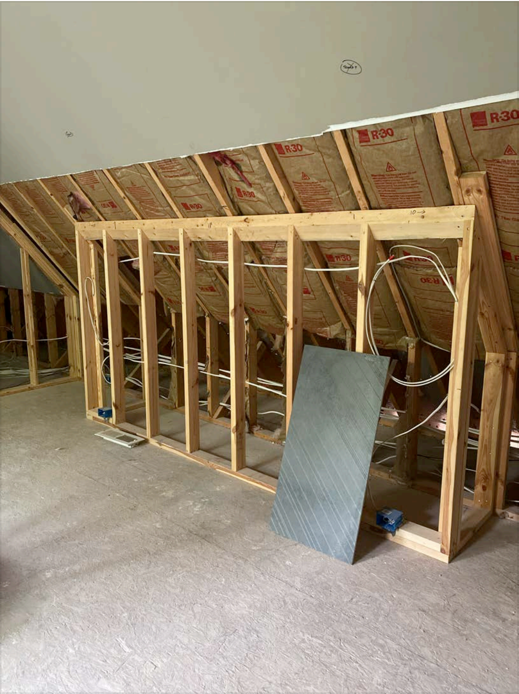
Room closet wall: 1 partial 2x8, 19 2x4
