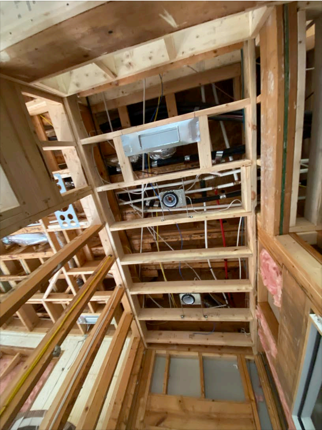
7 2x6 ceiling in garage entrance hall
