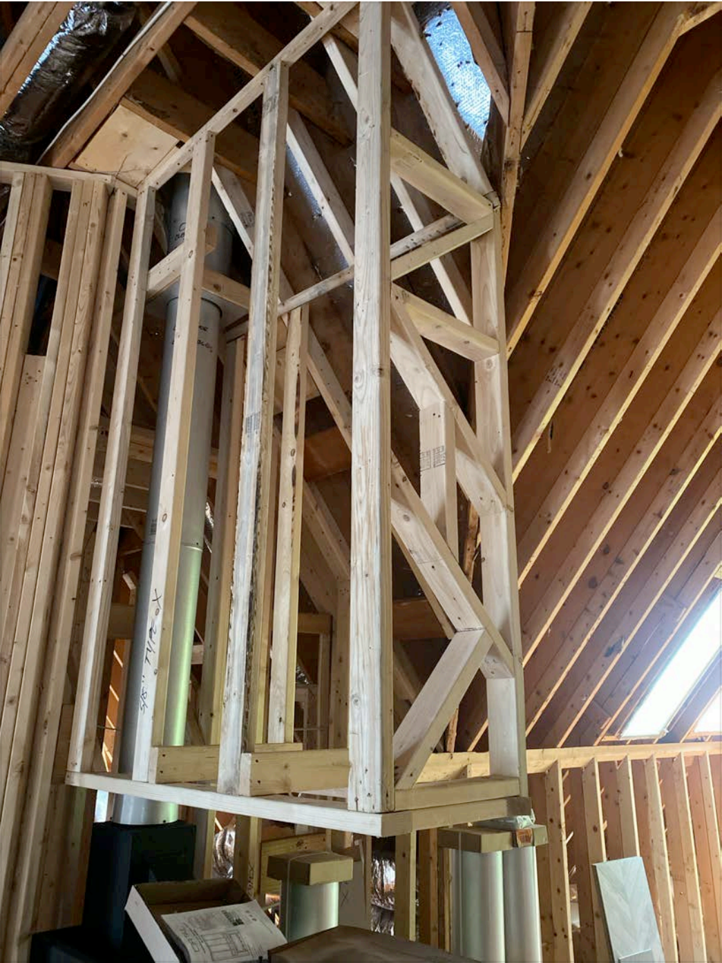
Tape lighting framing: 8-16 2x4
