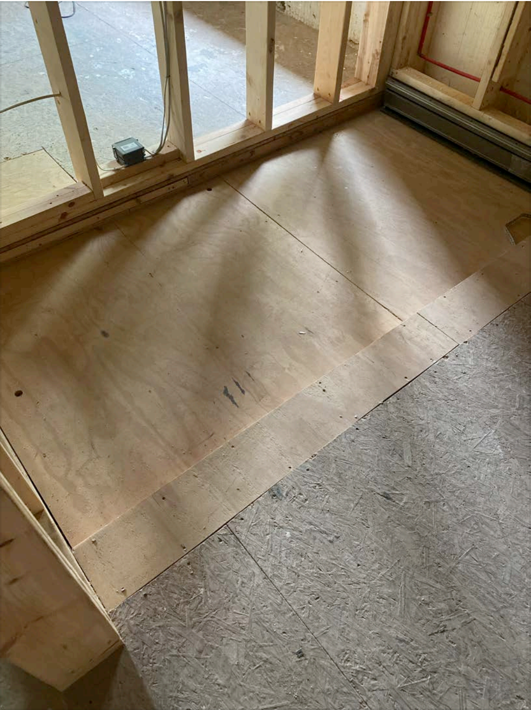
Under art room floor reinforcement (ceiling of master bedroom)
