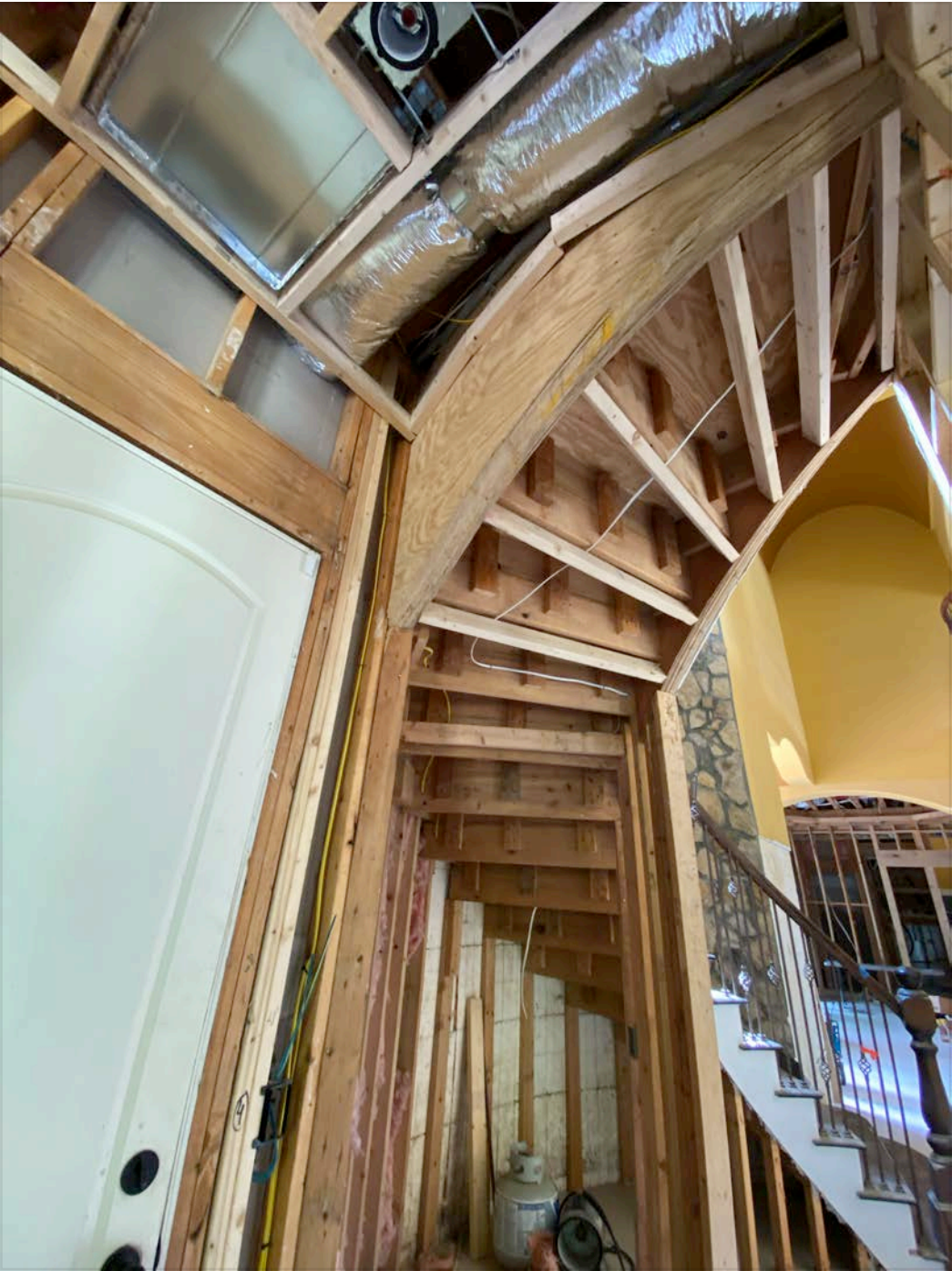
5 2x4 for area under stairs and alongside door.
