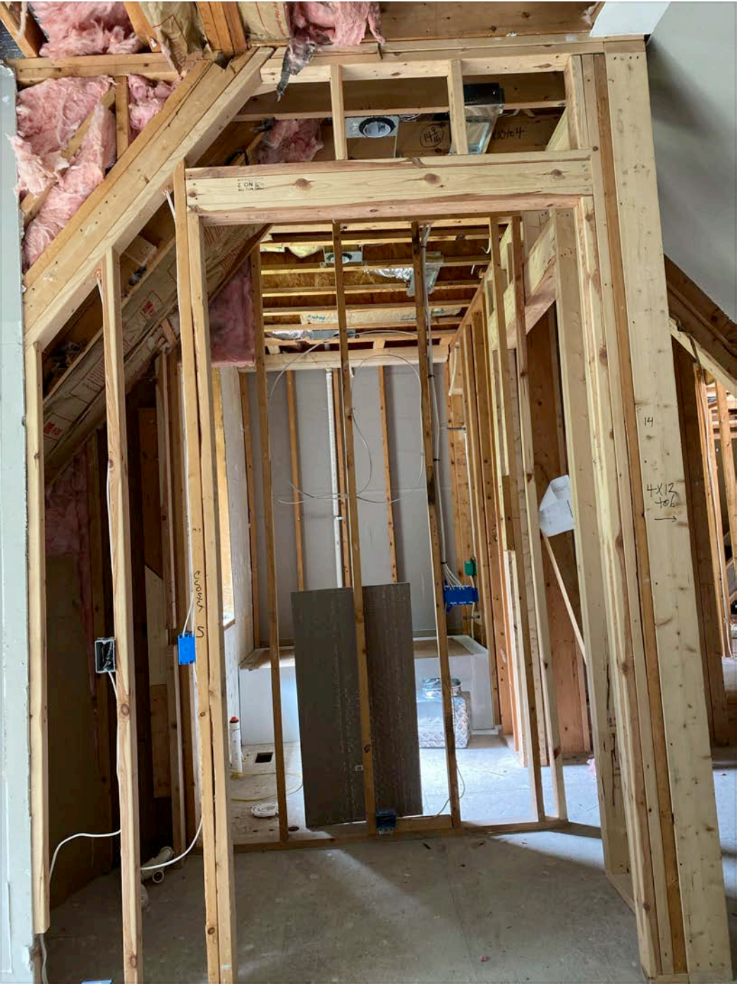
11 2x4 wall into closet
