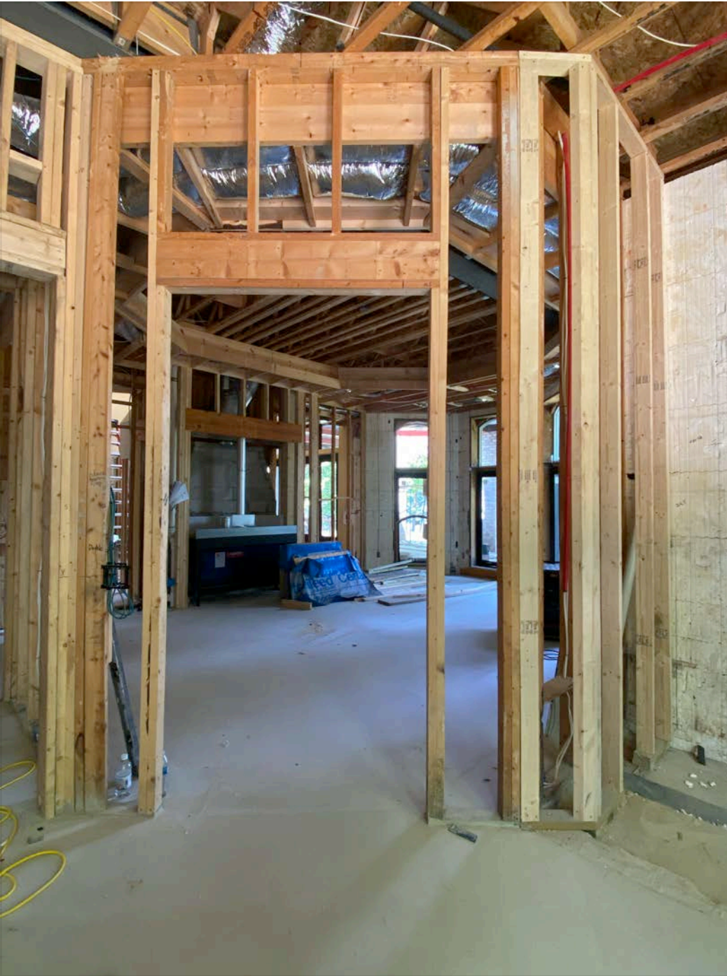
5-9 2x4 and reused header
