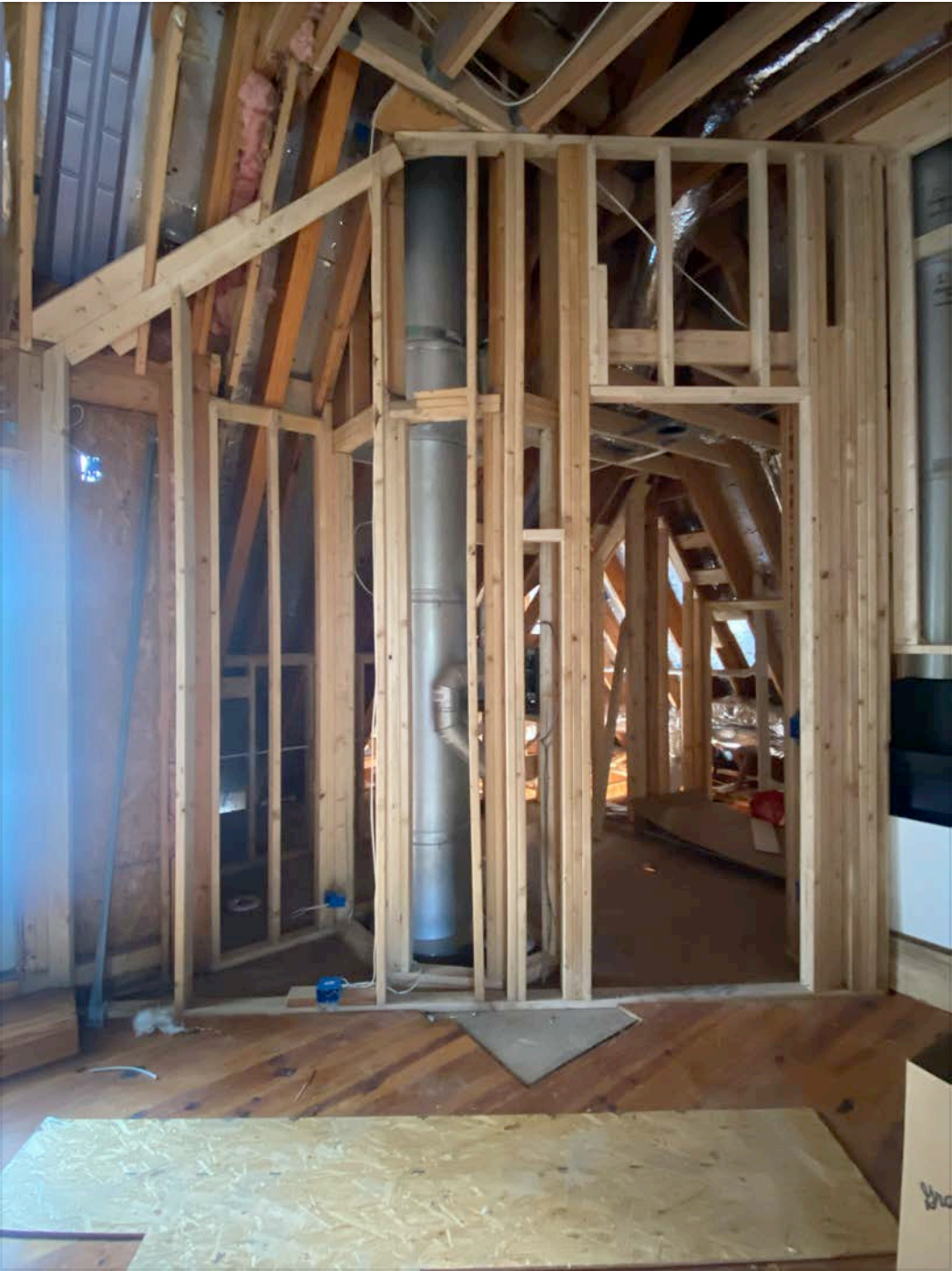
Bathroom back wall 11 2x4
