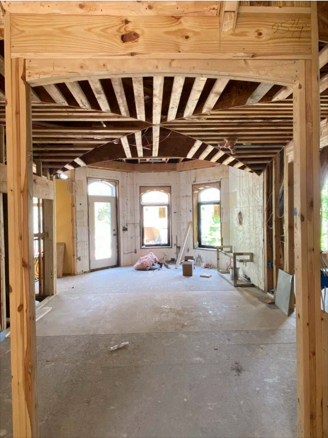
Fireplace wall reinforcement 12 2x4
