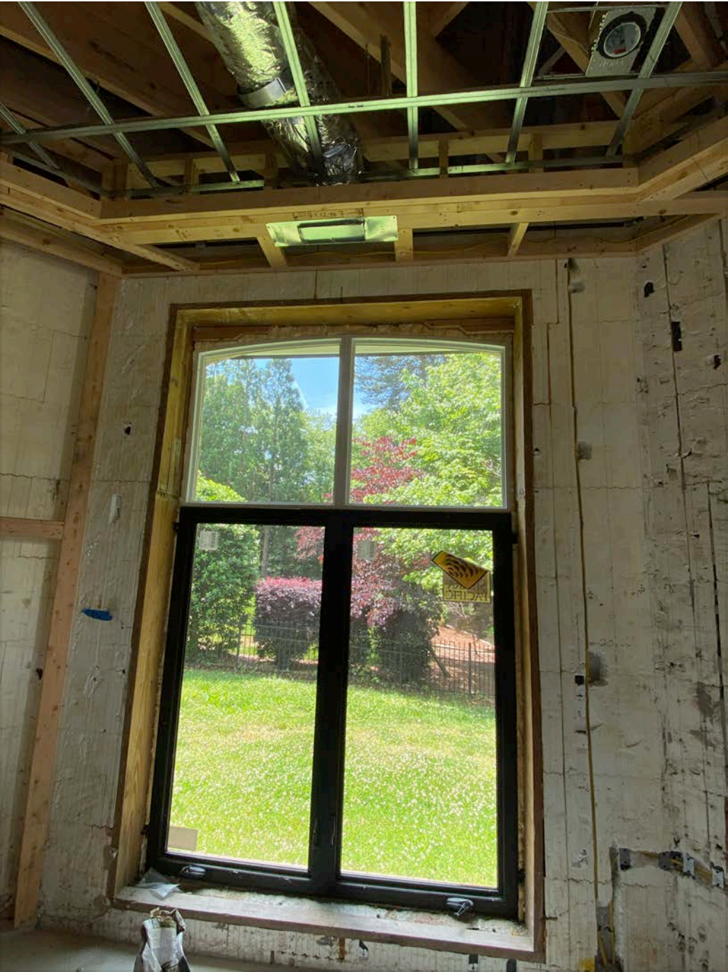
Keeping room edge work over window 7 2x4
