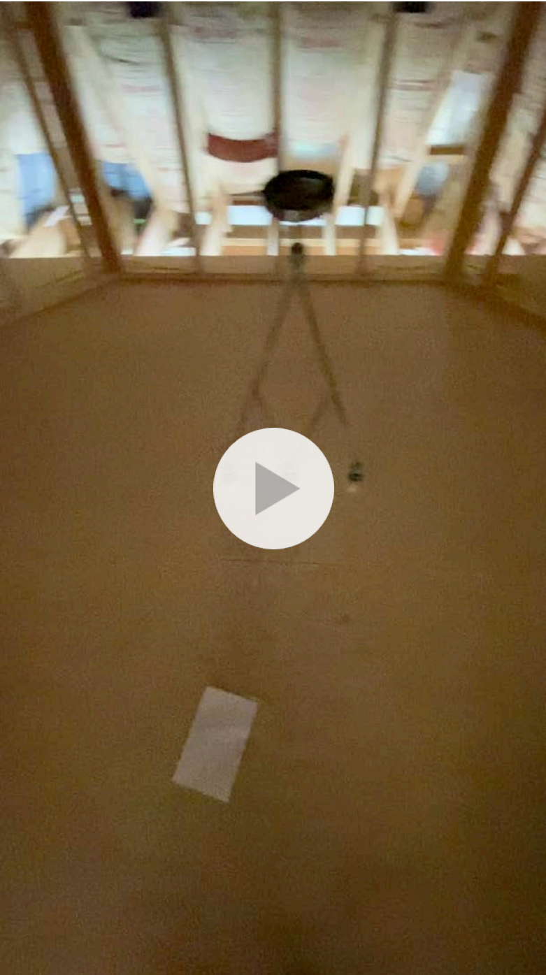
2nd level Elevator shaft floor:
