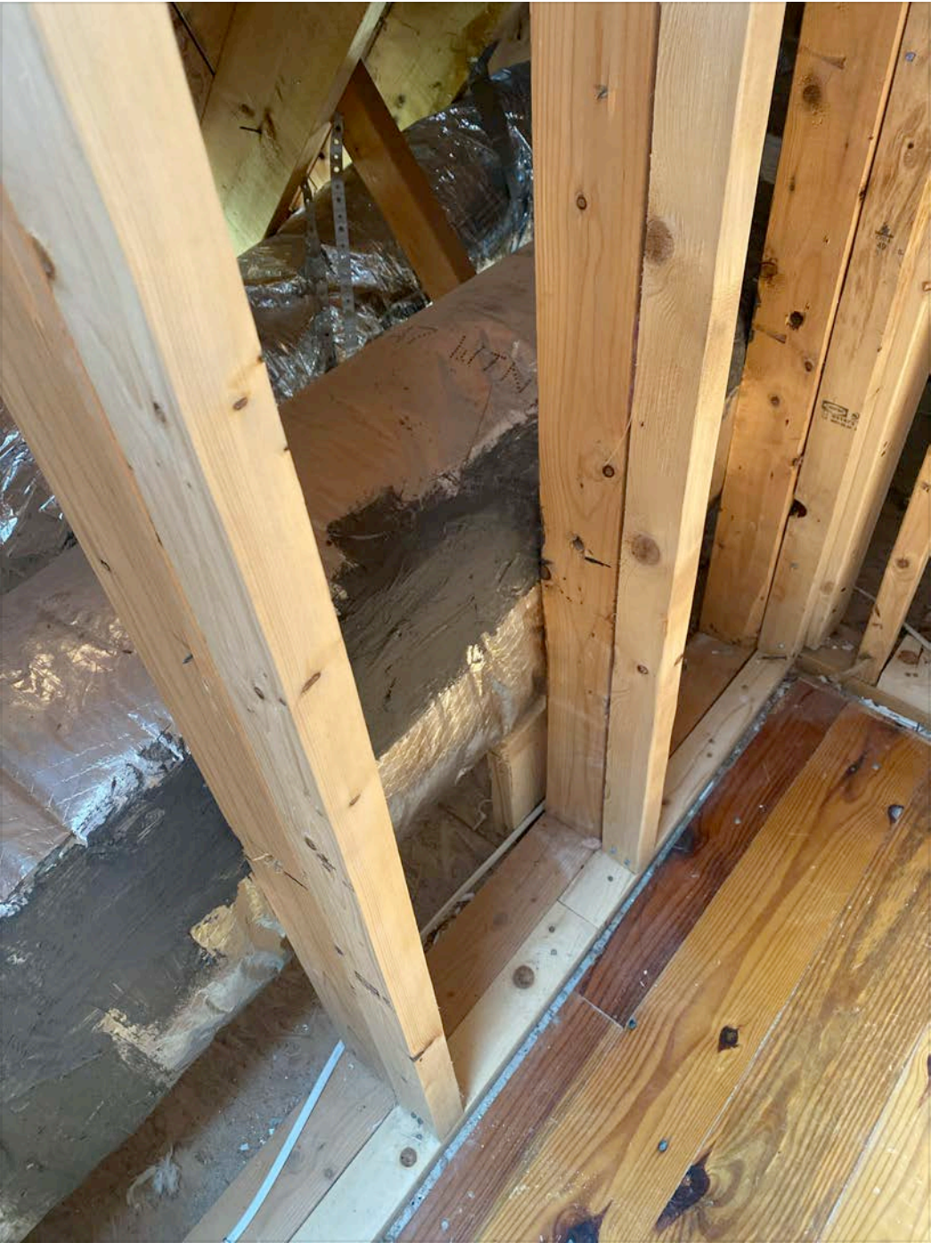
Fireplace base framing sheathing and 2 2x10
