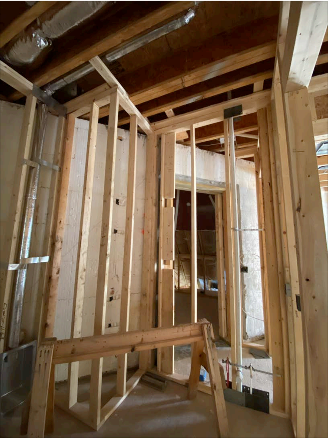
Chris' office entrance 10 structural 2x6 under beam
