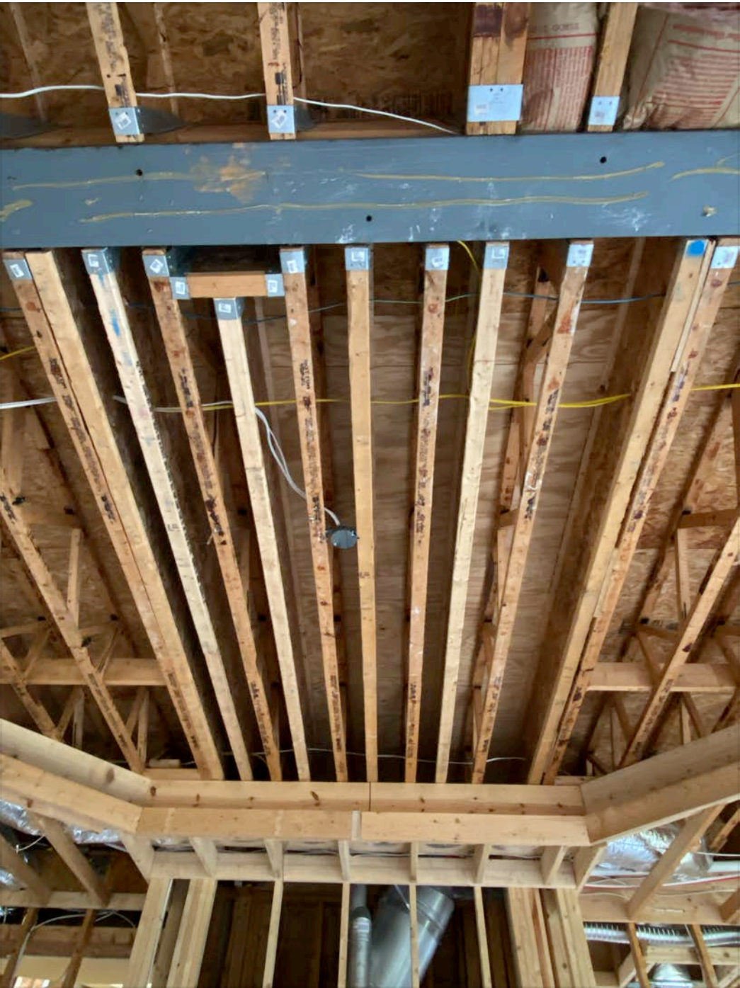
Shown from two perspectives above. 10 2x4, sheathing, and metal brackets.
