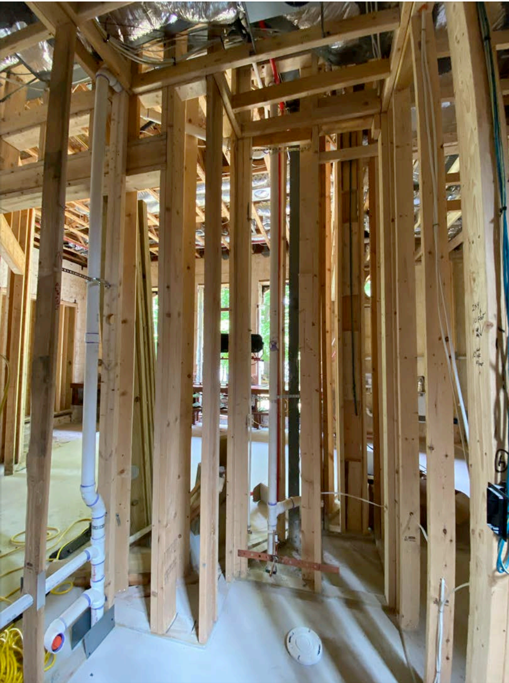
END OF FIRST FLOOR FRAMING (Less than 400 boards)
