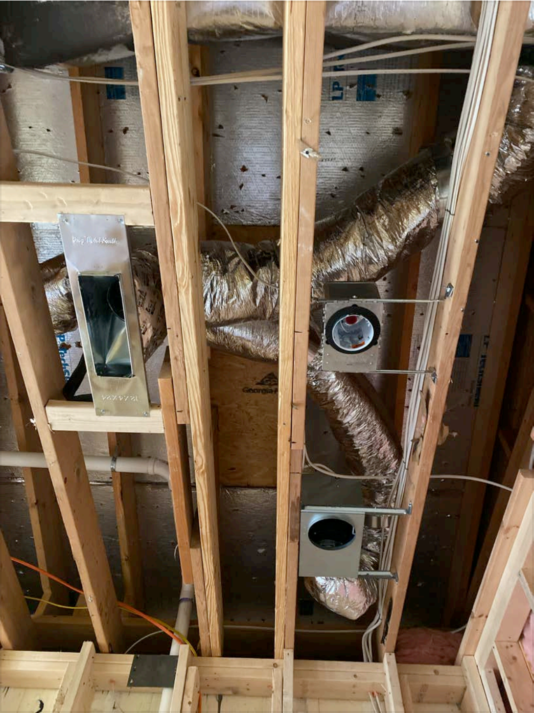
Guest room partial wall and entrance, shared with utility room: 17 2x4 and 1 2x6
