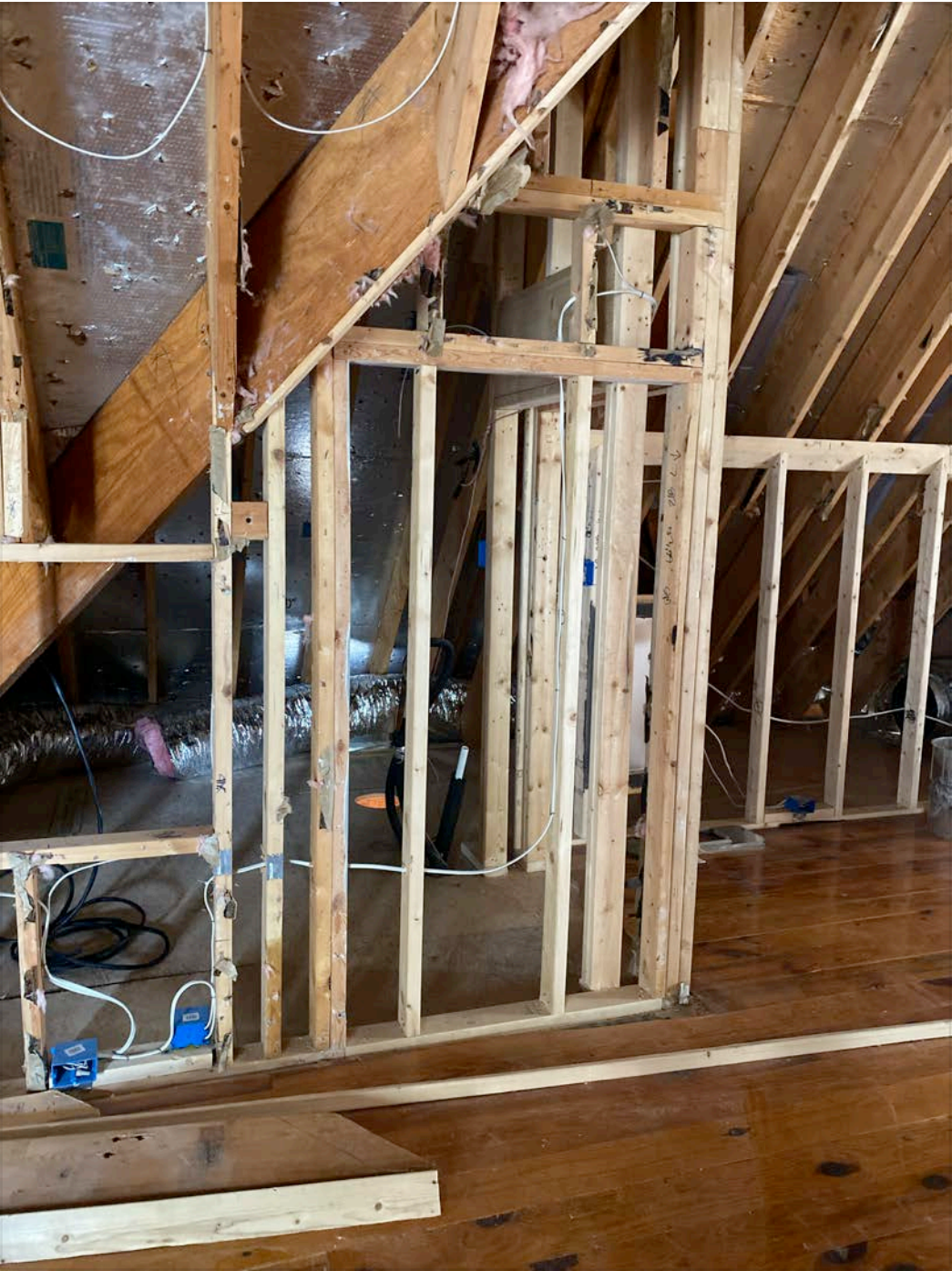
Framing opening new utility entrance point 13 2x4 and one 2x12
