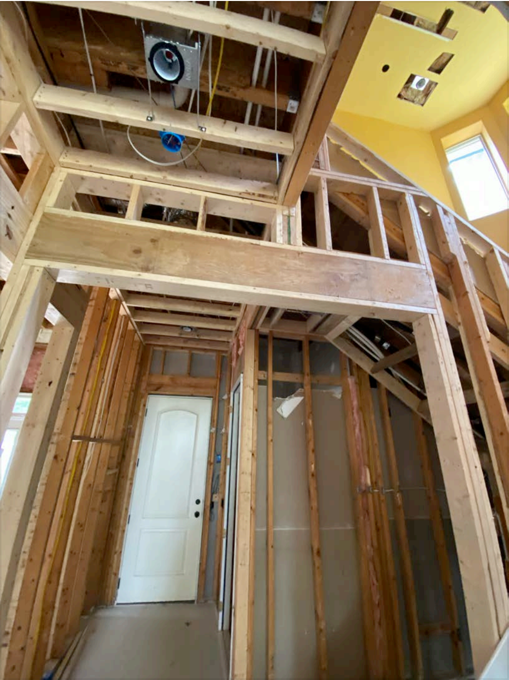
Reused two 2x12 8' wood for header (old and muddy)
