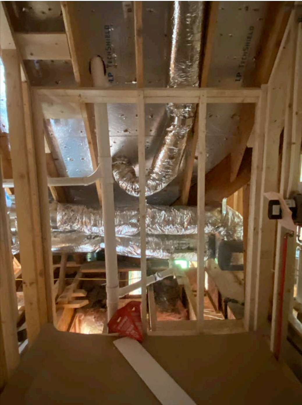
7 2x4 for reinforcement of shower remaining wall
