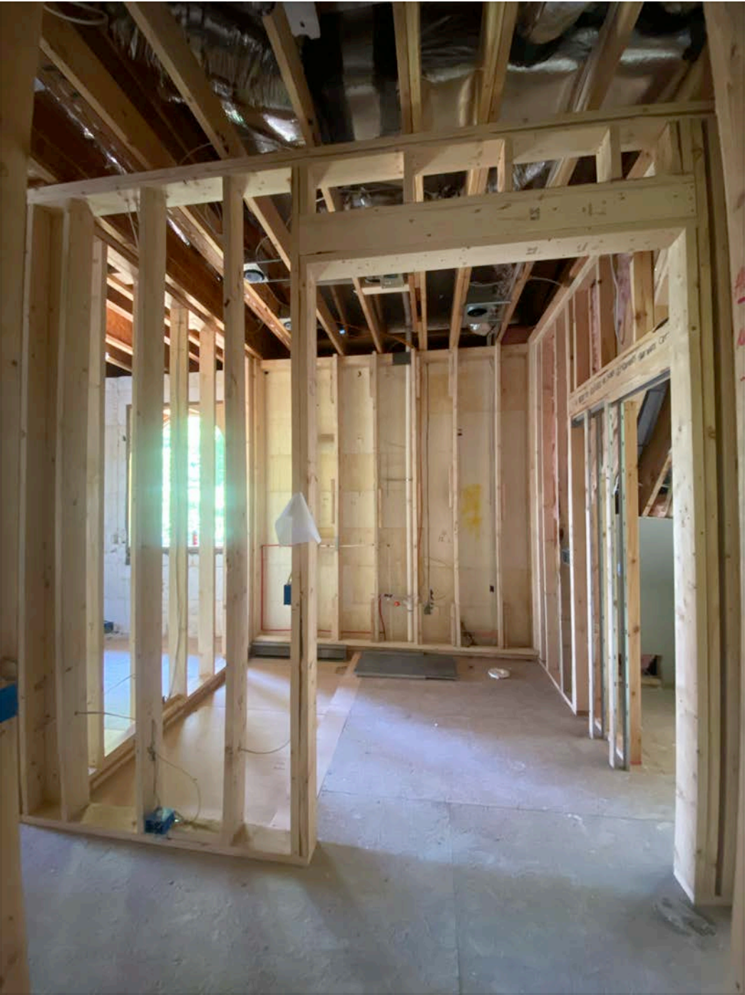
utility wall in hallway: 14 2x4
