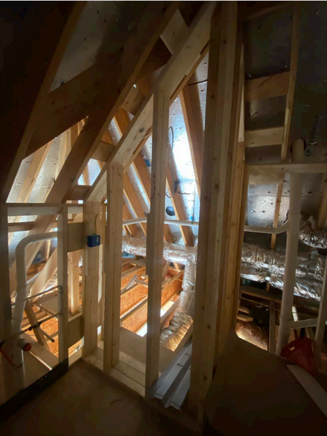
Fireplace structure walls:
