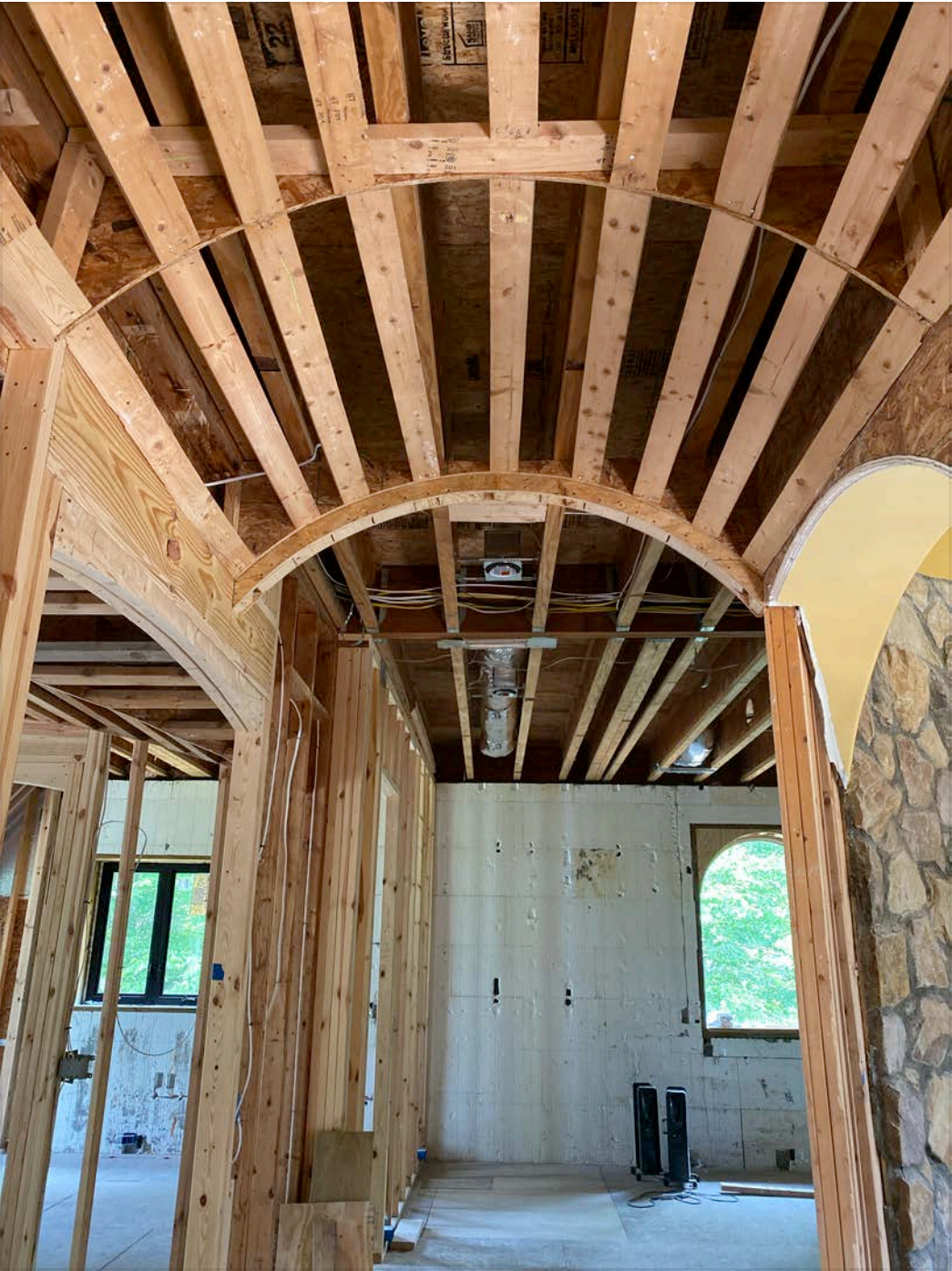
Doorway with header: 7 2x4 and 2 2x6 and 2 2x10
