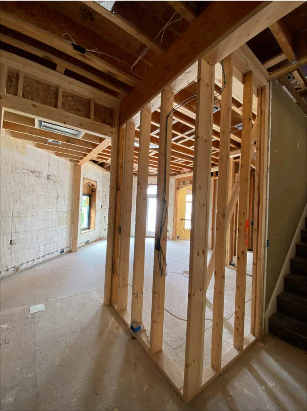
Goes with 4 new 2x4s to support load across hallway
