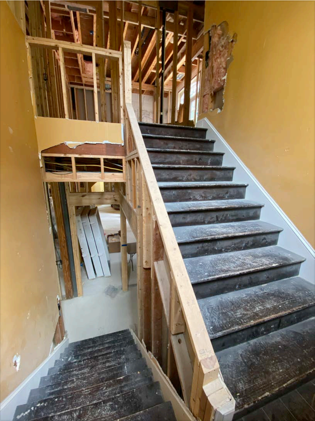
Stair area some temporary 5 2x4
