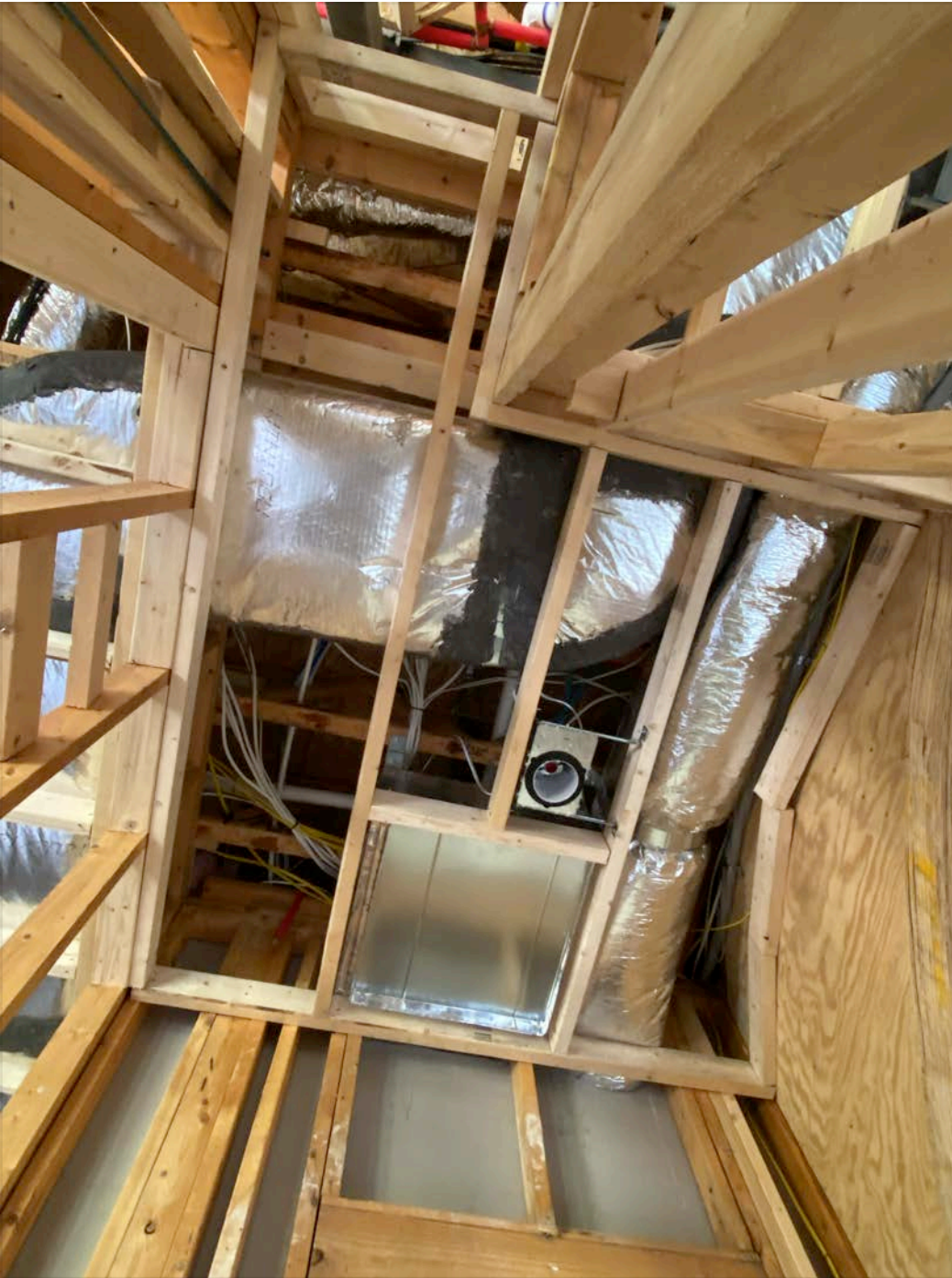
8 2x4 ceiling upon entry to house from gym
