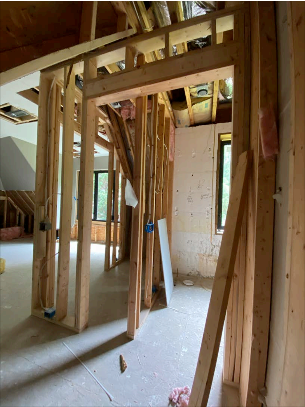
Bathroom door wall 13 2x6 including header
