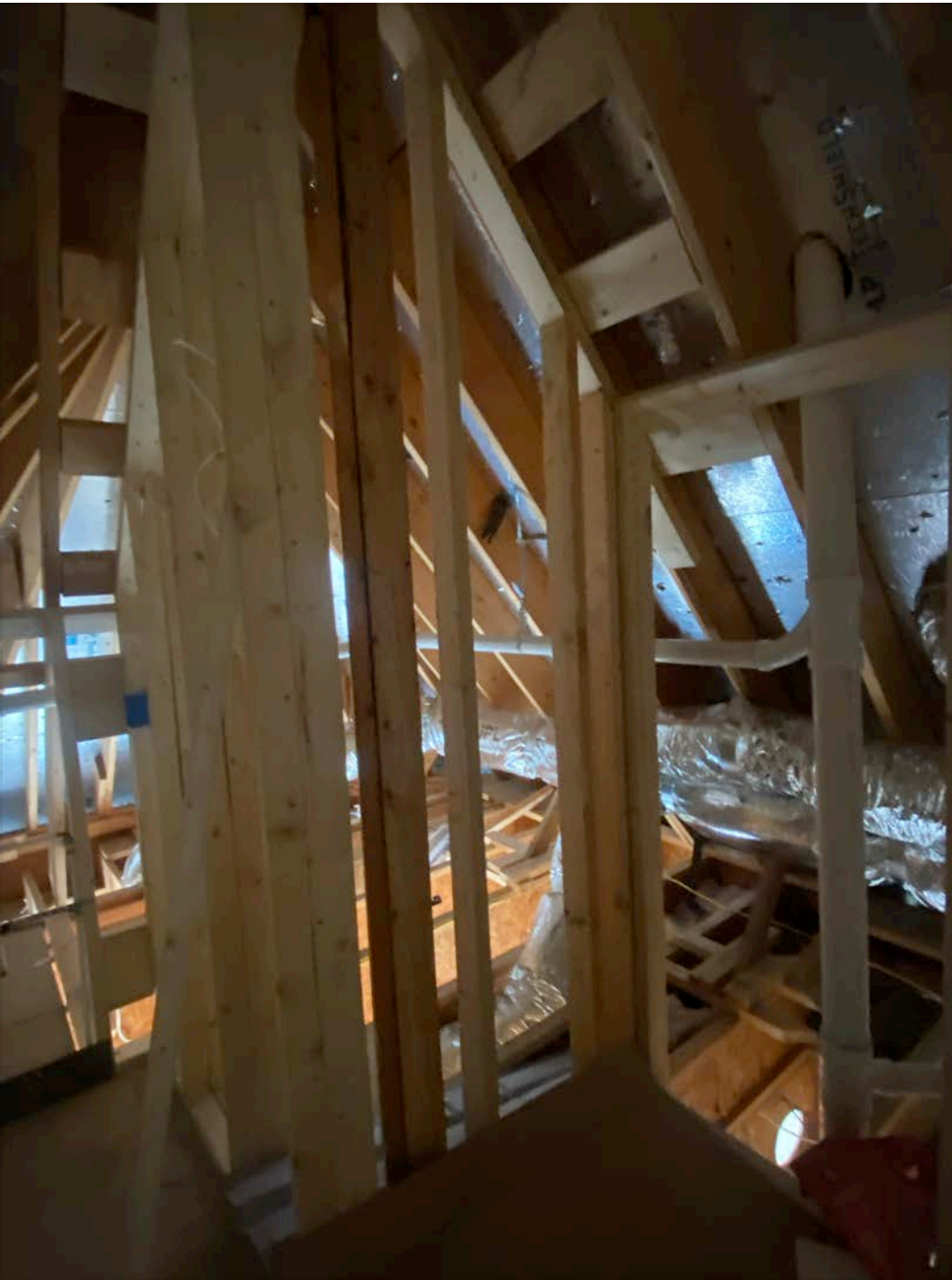
11 for mid-framed remaking wall
