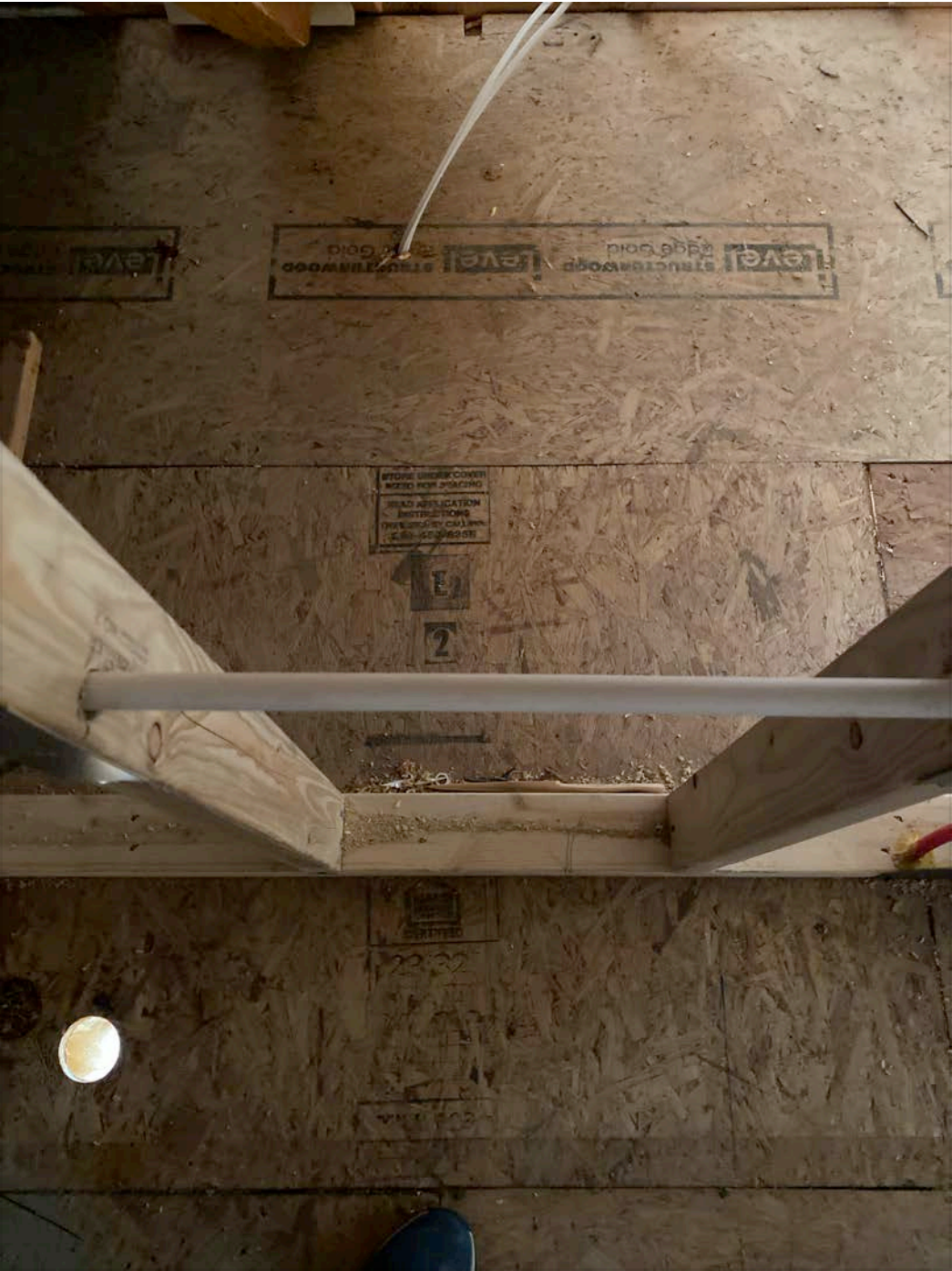
One in third floor elevator shaft closet (cut portions placed together)
