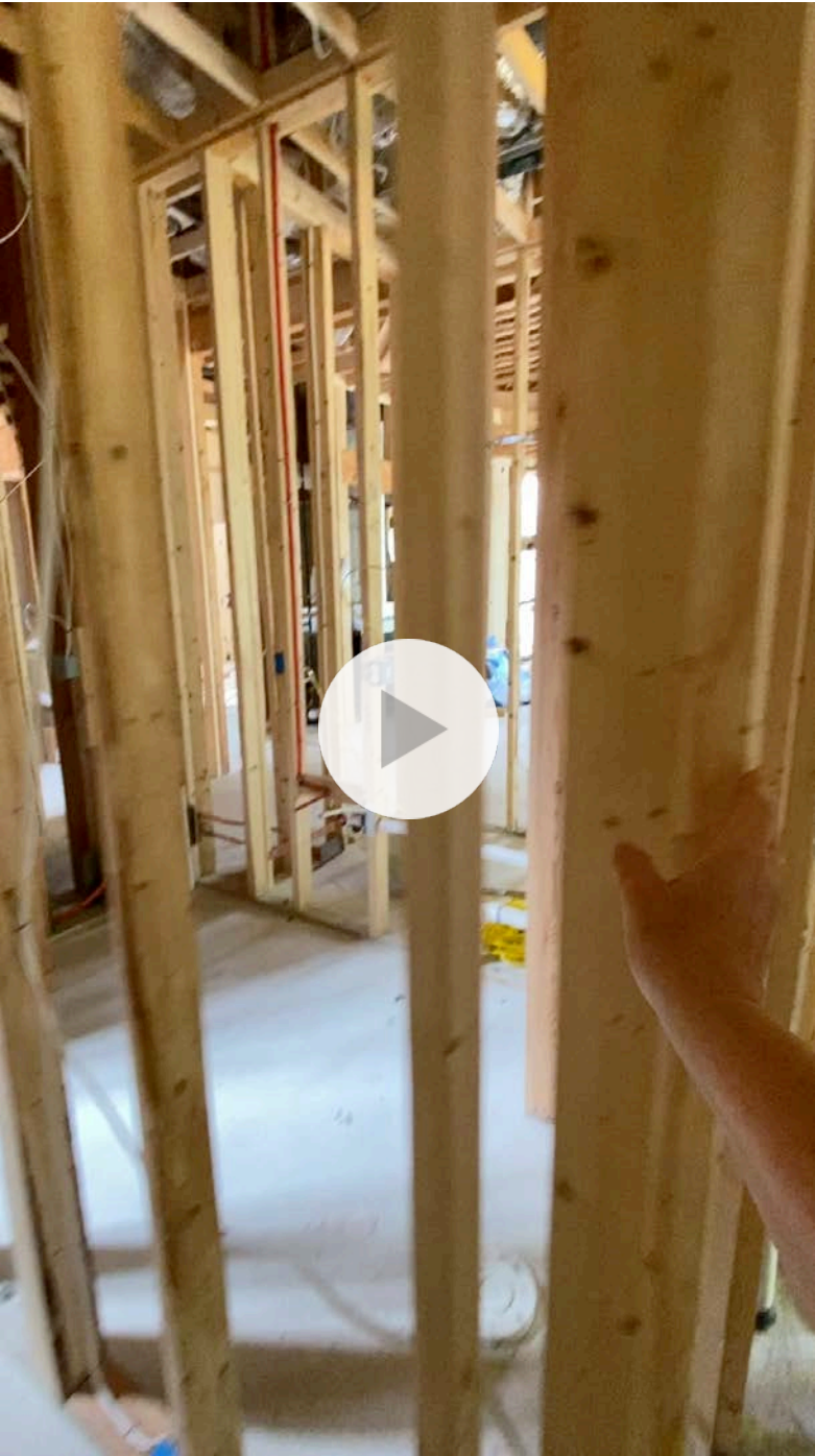
8 2x4 for sink wall
