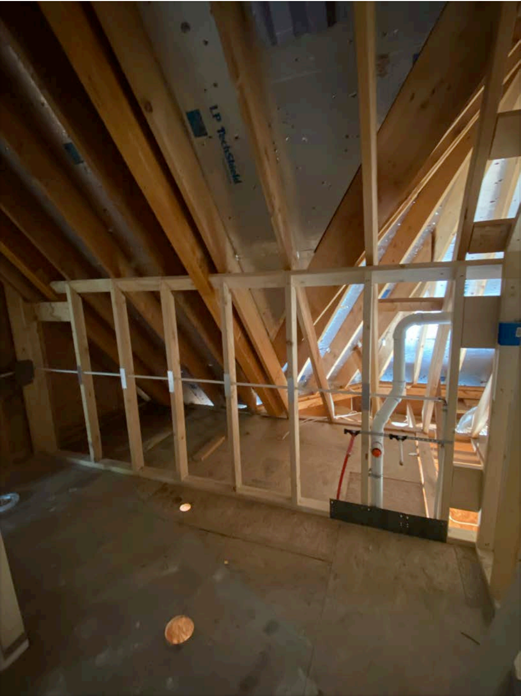
Shower wall 12 2x4 on shower trim wall
