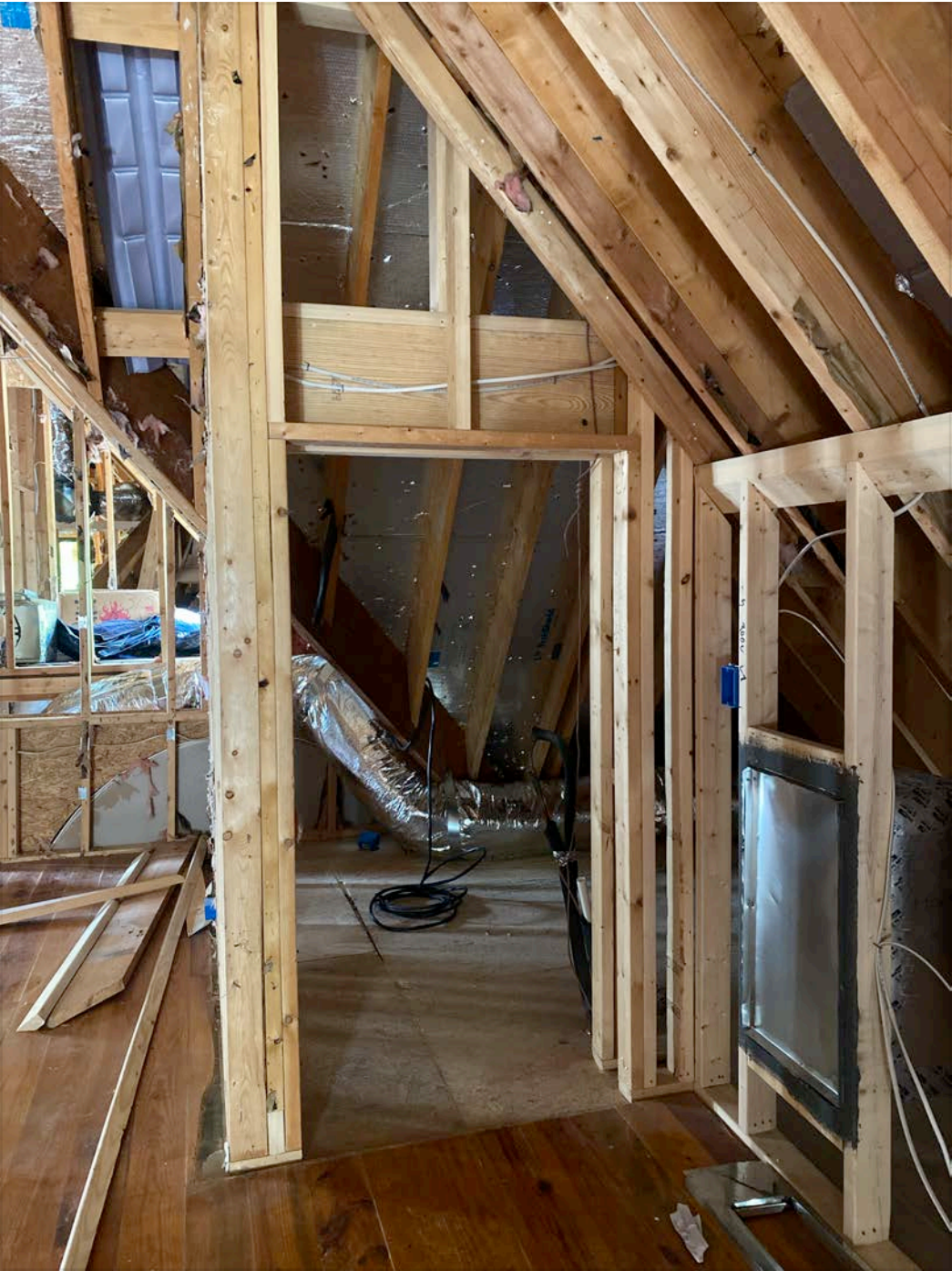
Evening of wall near elevator shaft
