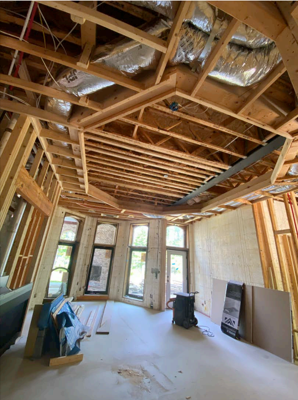
Frame around master bedroom ceiling
