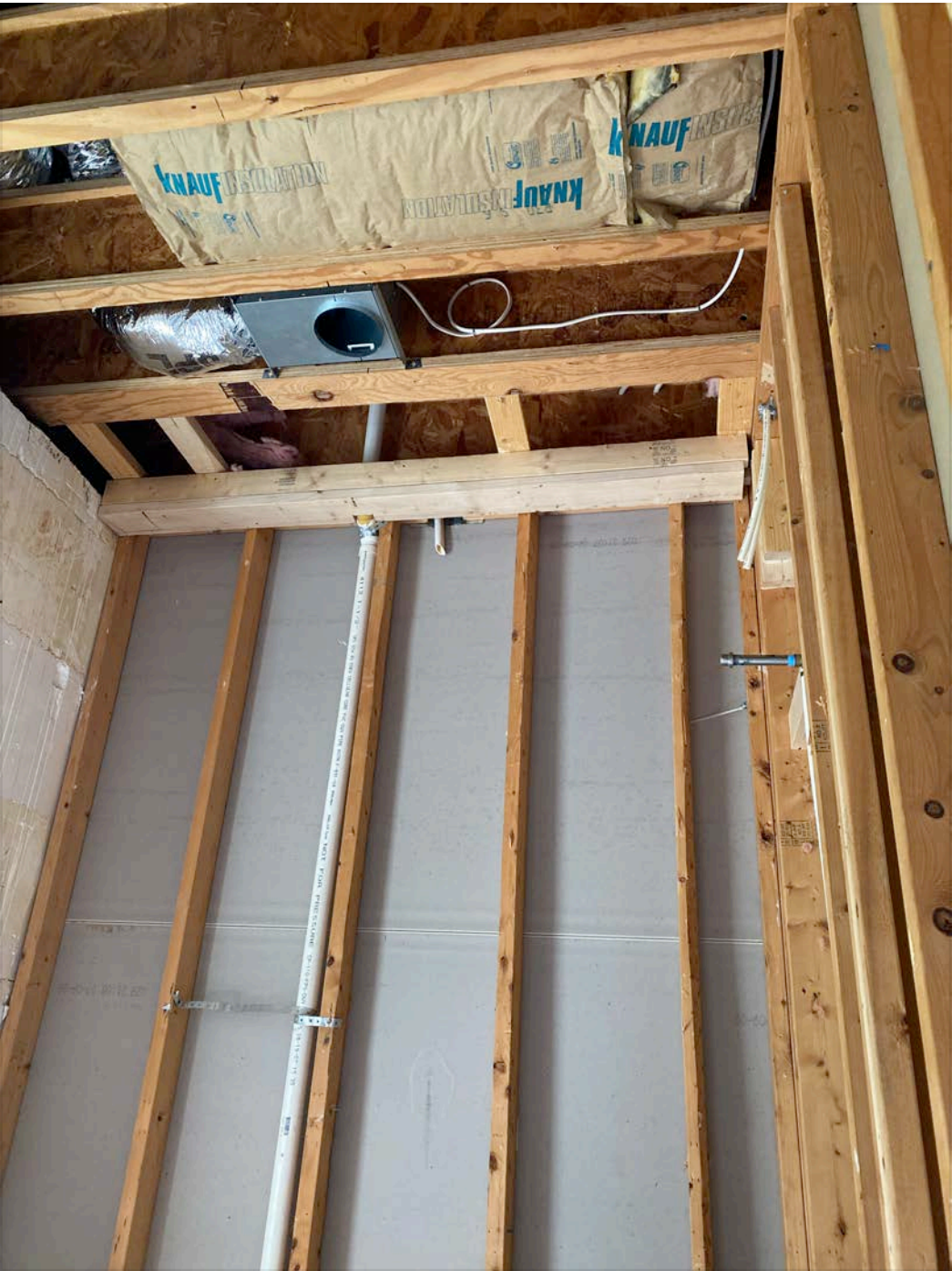
Pipe hiding wood 1 2x6 and 1 2x4
