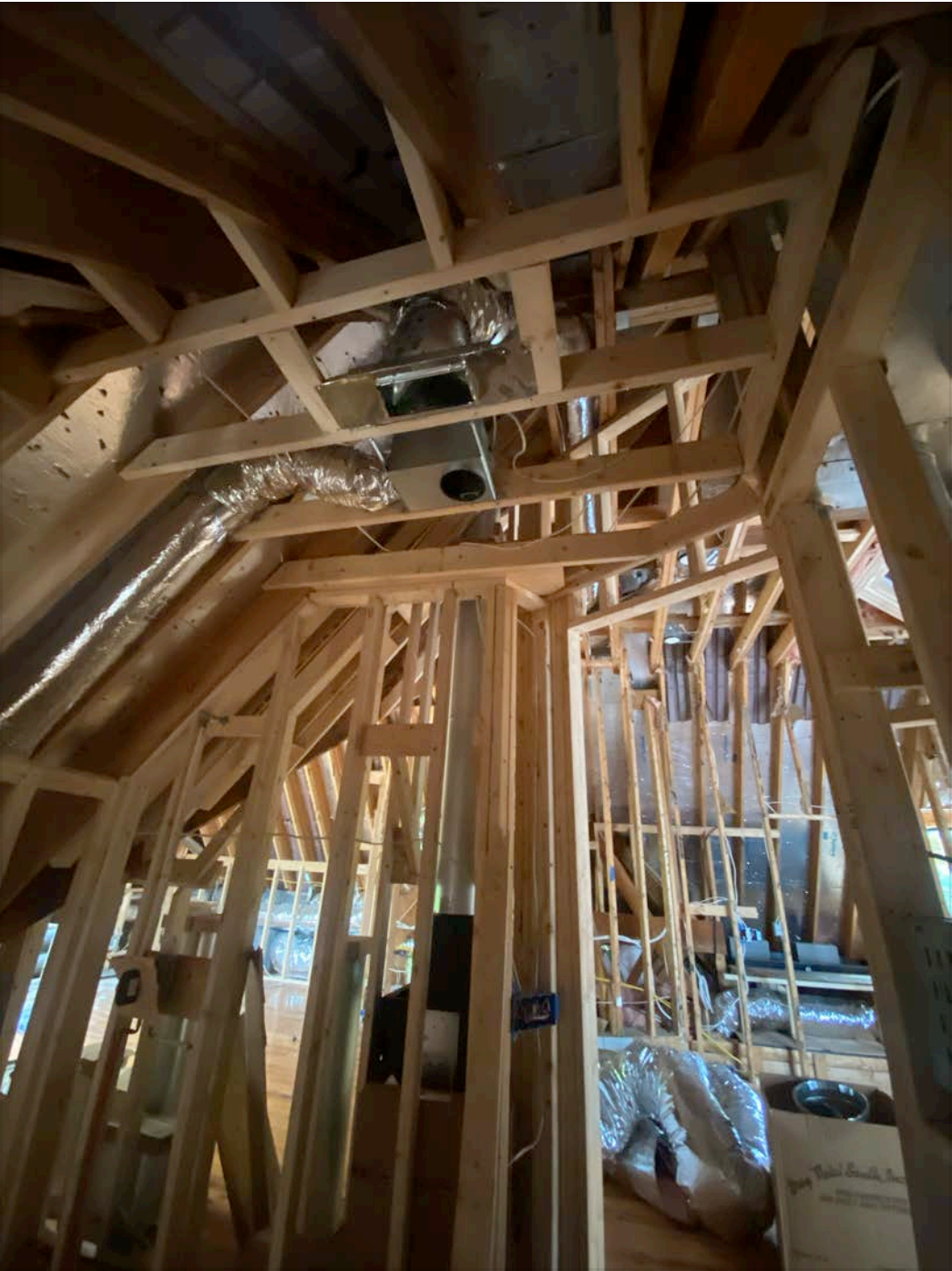
Framing to enclose of old utility door area: 2 2x4
