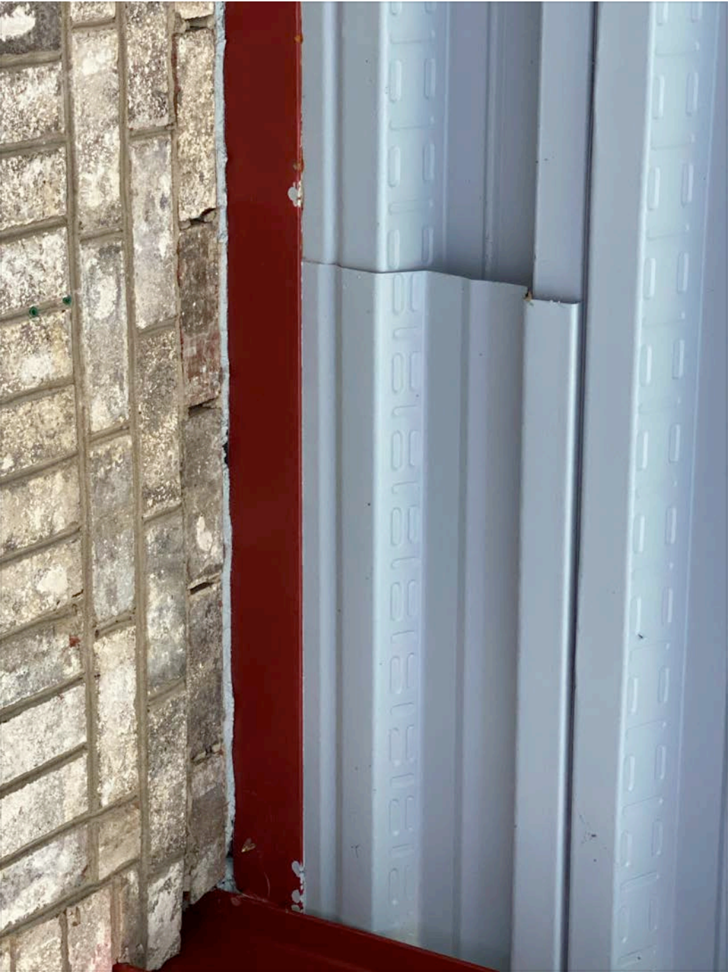
Window measurements off
