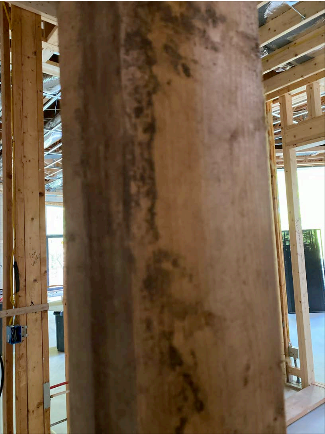
Salvage header used in entry to powder room
