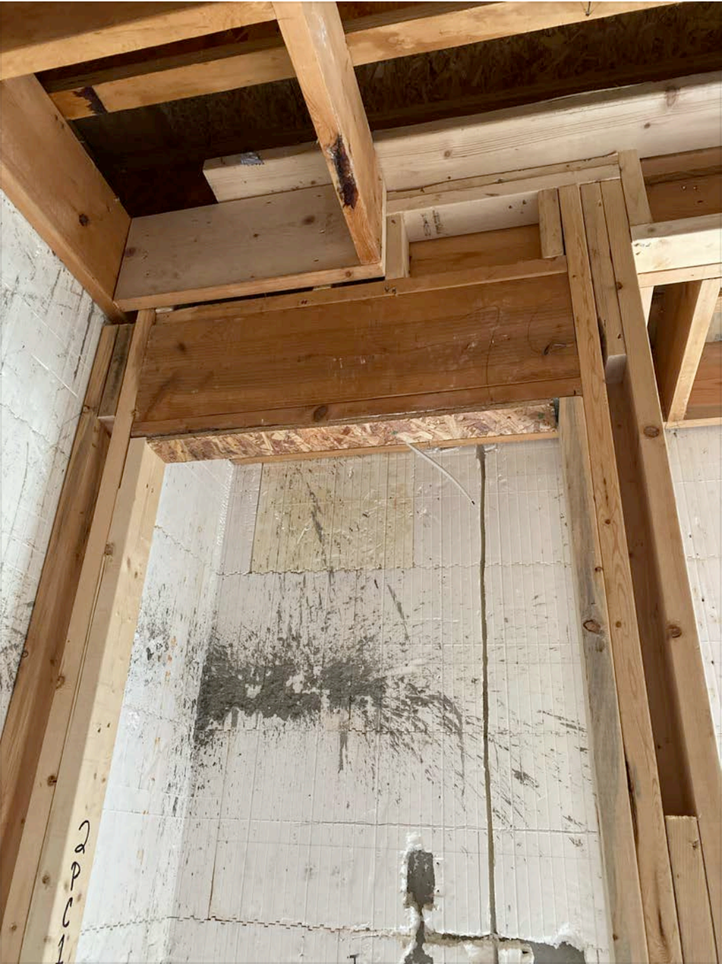
Muddy salvage header installed in mud room entry:
